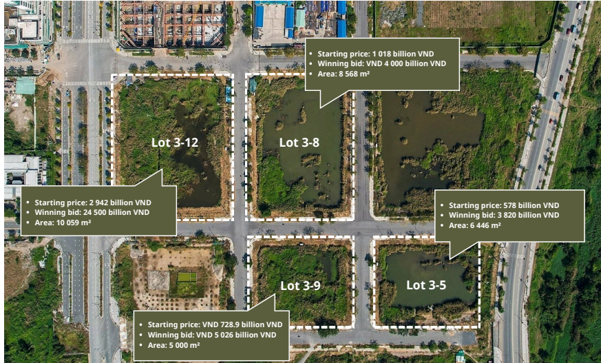
Figure 1: Four land plots in the 2021 Thủ Thiêm auctions. The aerial view details zones 3-5, 3-8, 3-9, and 3-12, which were subject to speculative bidding and default. Source: Adapted from Lao Dong Newspaper.
